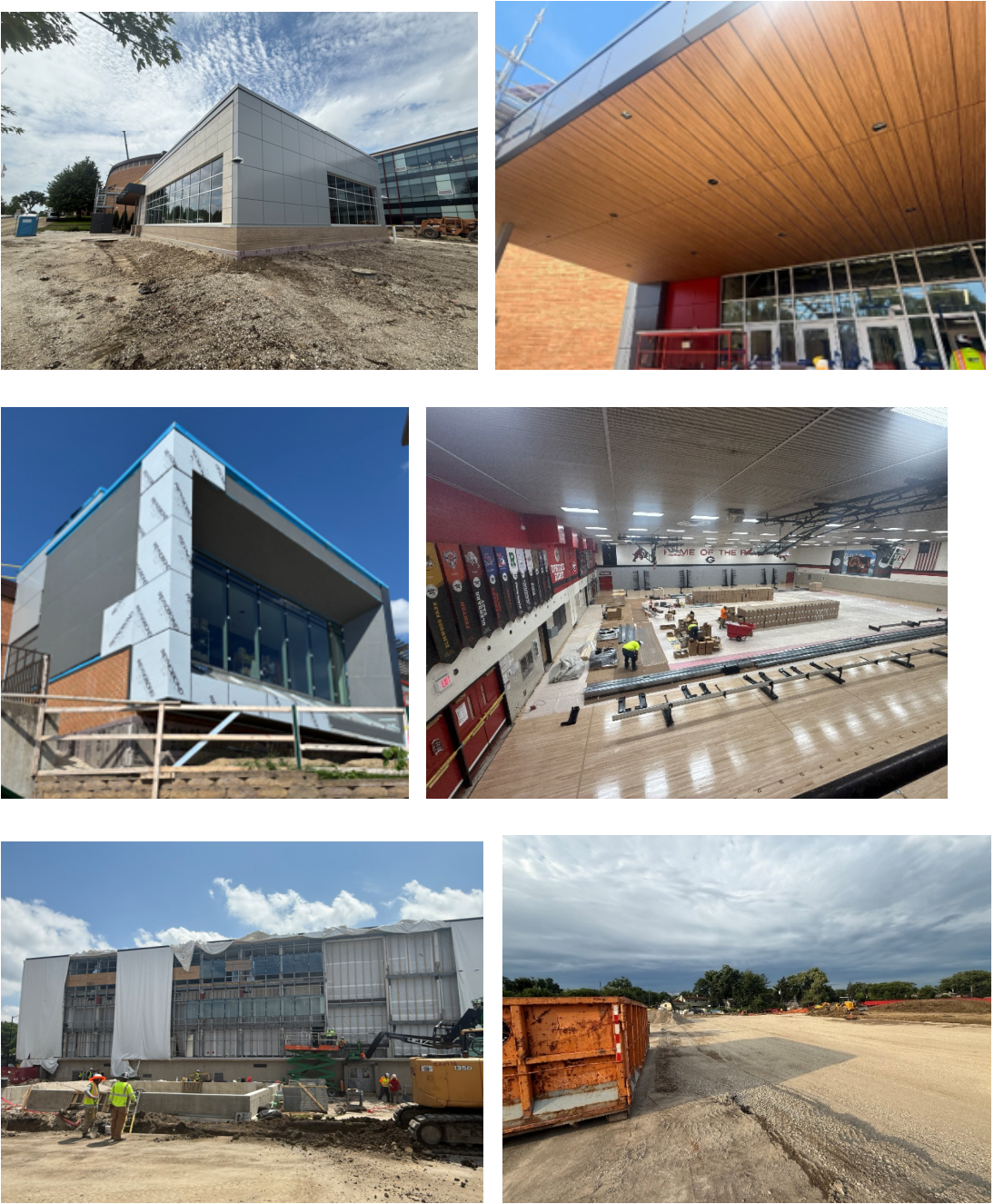
Phase 1 Phase 2 progress:
