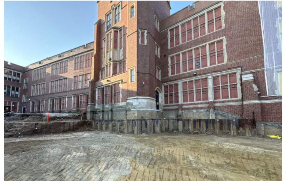
Excavation Following Earth Retention Install
