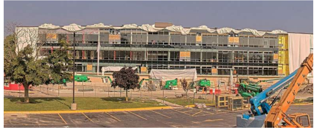
West Elevation Curtainwall Replacement
