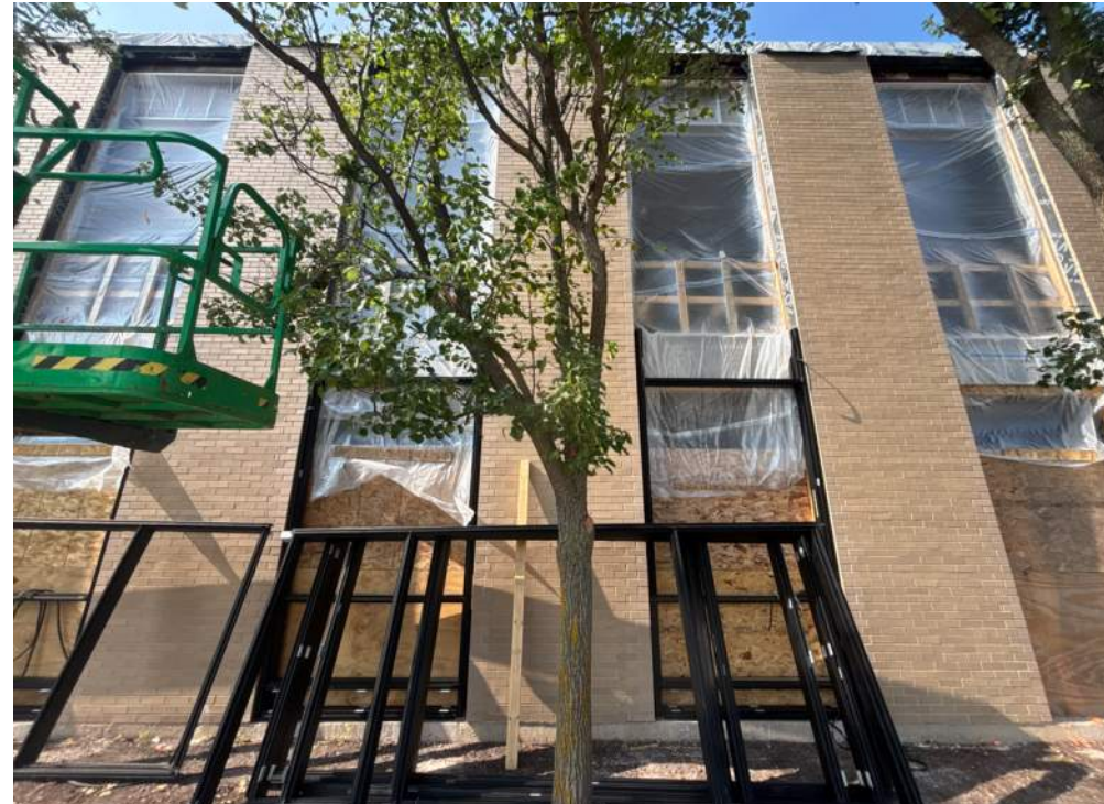
New Window Installation
