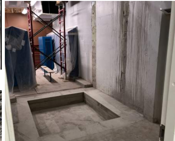
LULA Elevator Pit Created
