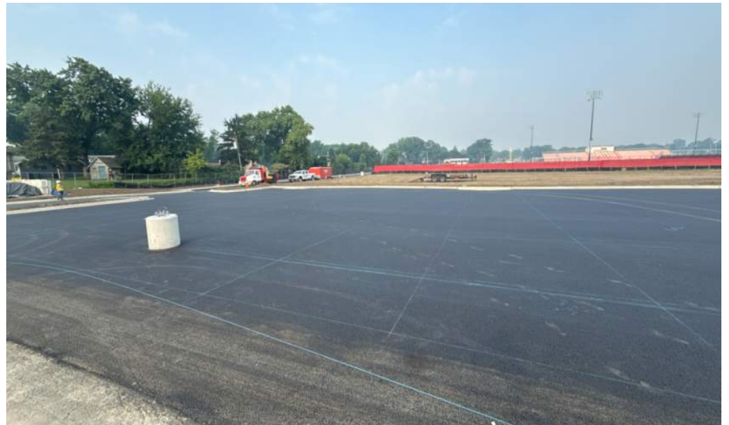
New Parking Over Storm Detention System
