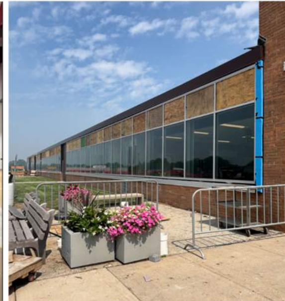
South Window Replacement
