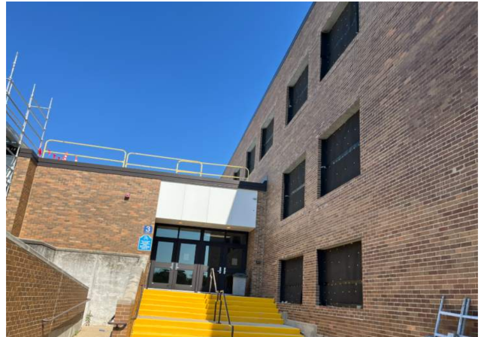
New Window Openings Created
