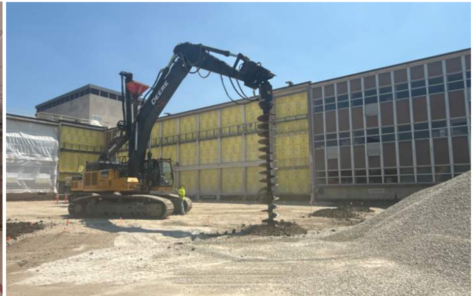
Learning Commons Rammed Aggregate Pier Install
