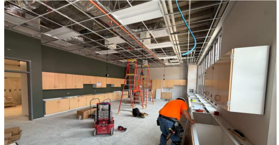
Science Lab Renovations
