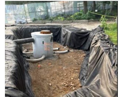
Drywell Installation for Stormwater
