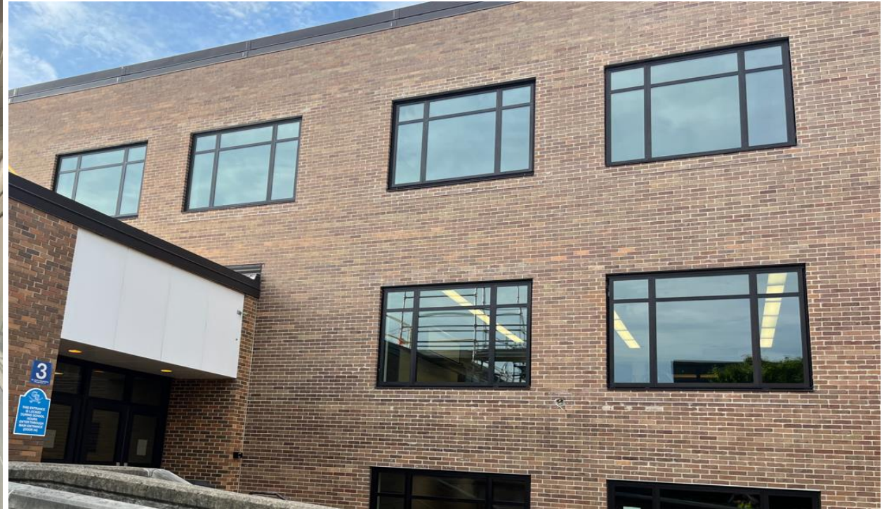
New Windows Installed
