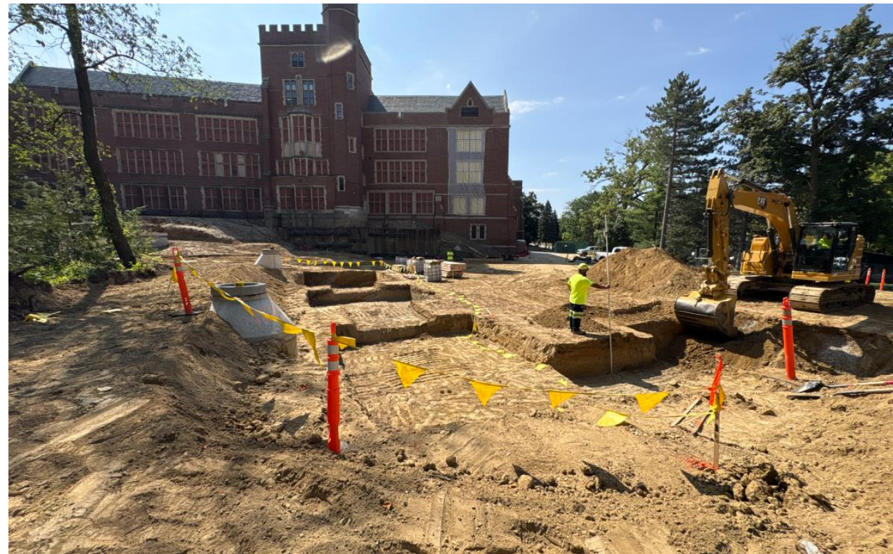
Classroom Wing Footings In Progress
