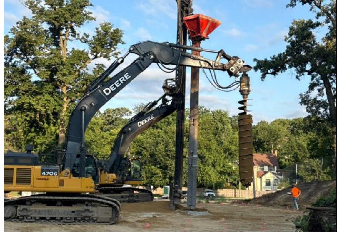
Rammed Aggregate Piers Installed
