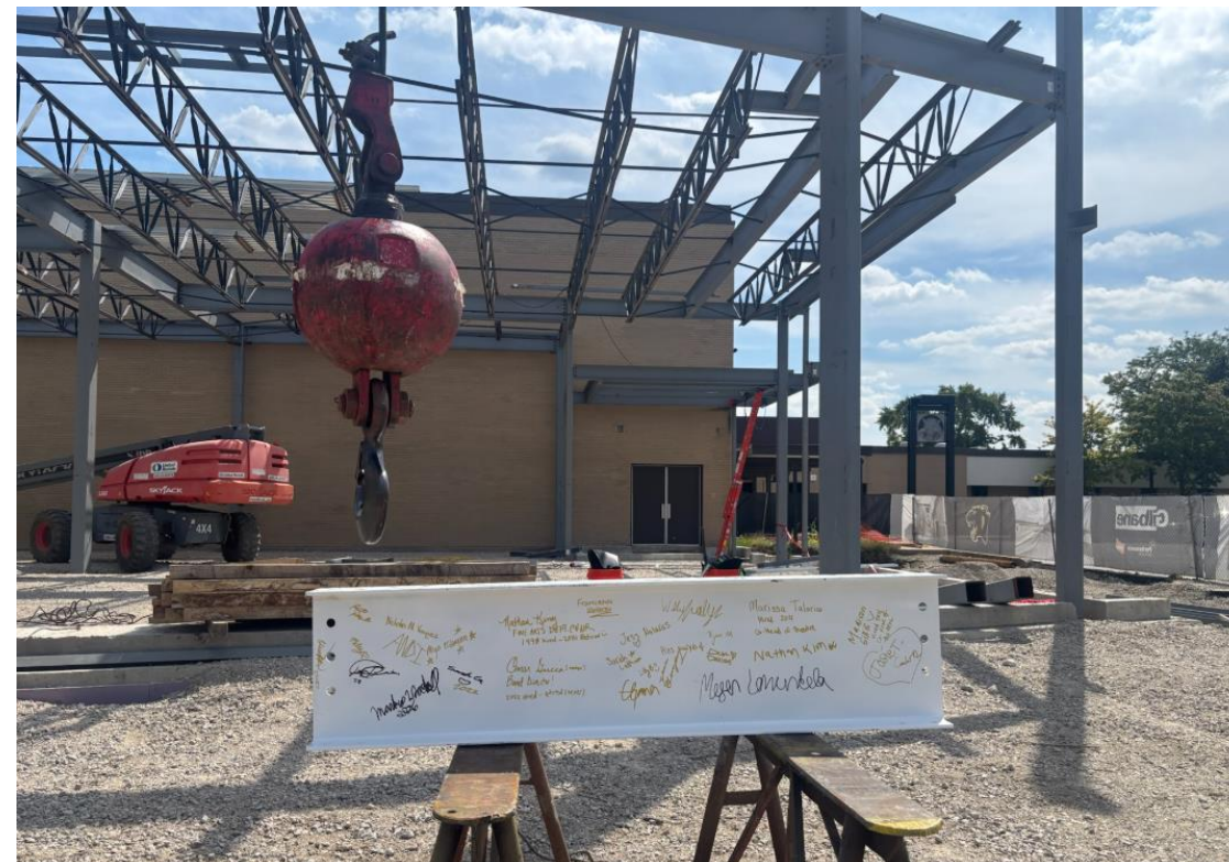
Music Addition Structure Topped Out
