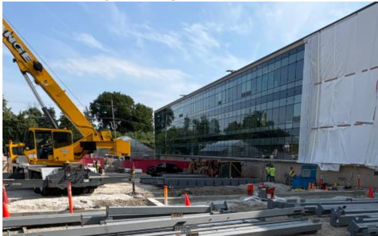
West Curtainwall Replacement
