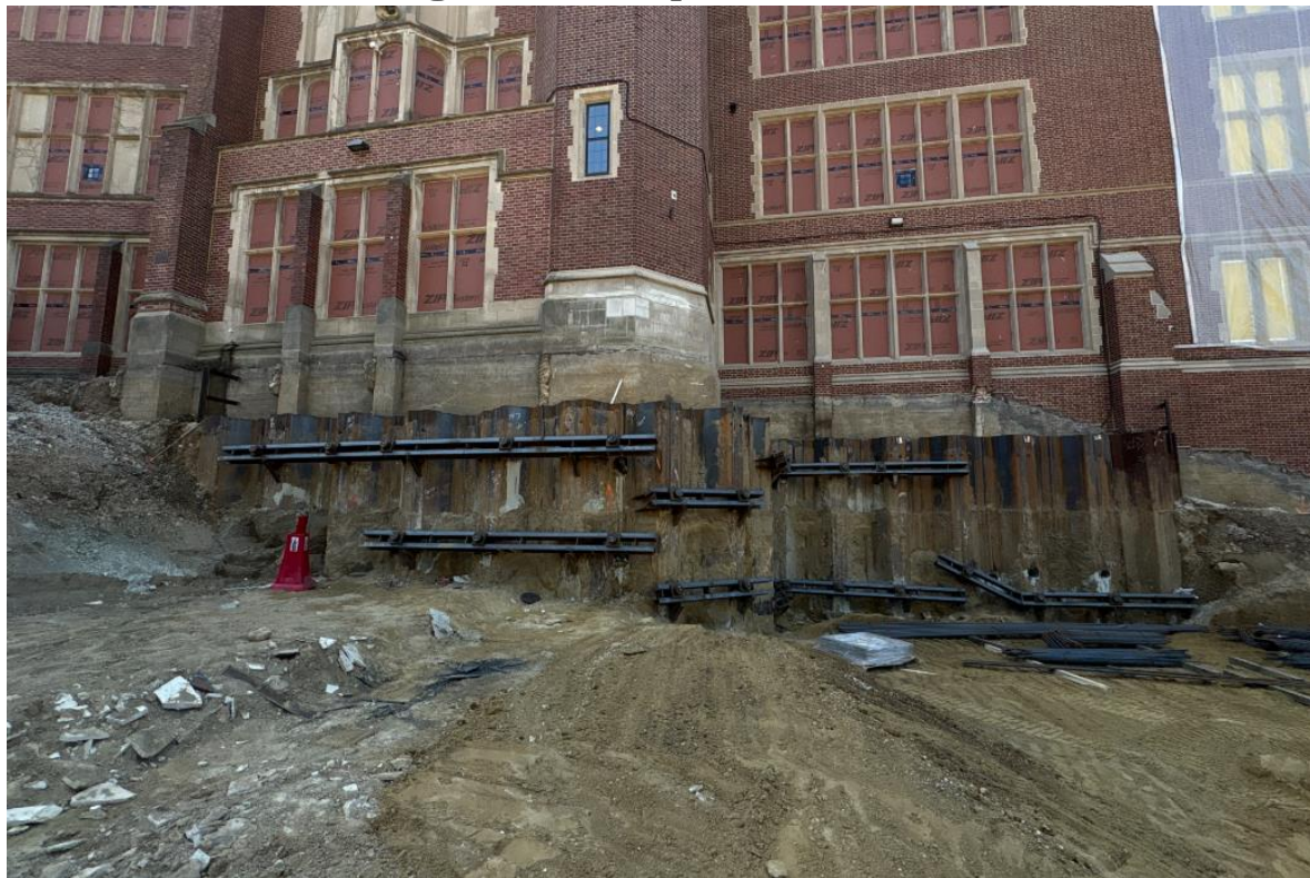
Earth Retention System Complete
